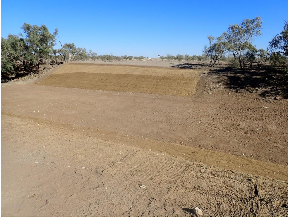
Figure 1: Example of reinstated bank for watercourse crossing at KP431 (29 July 2018)
