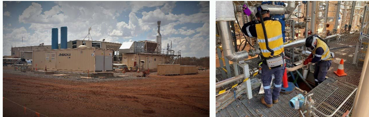
Crews performing key maintenance works at Jemena's Phillip Creek Compressor Station
